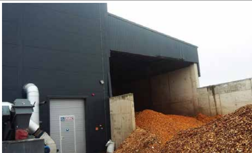
Picture 1. Woodchips before entering the bunker. (Photo: Vidmantas Verbyla)
